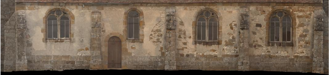
Figure 4: A typical orthoimage generated by orthographic projection of a dense point cloud.
